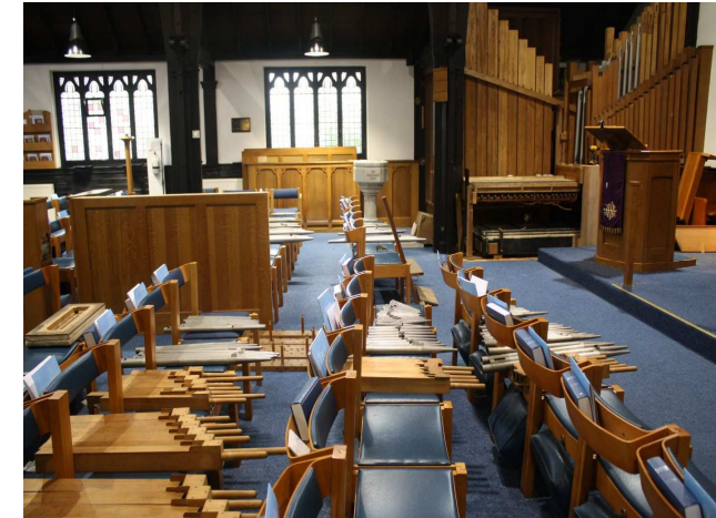
All the pipes removed and laid out on the chairs
