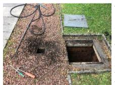
There was no other solution than to get Probe Drainage in to pump out the cellar again, which they arrived to do on 8th July. However before we started pumping I asked them to open the sump above the main sewer outlet from the whole site (the square manhole to the east of the path from the gate to the main door – see Fig 2). They found this flooded to what I judged to be the
